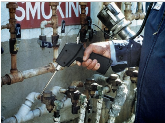
Test steam traps
